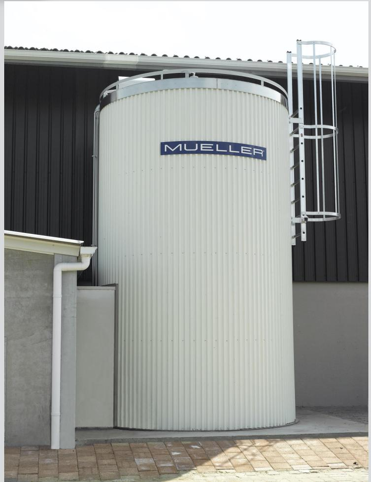
The silo is coated in a weather proof aluminium jacket in a 'off-white' colour.
